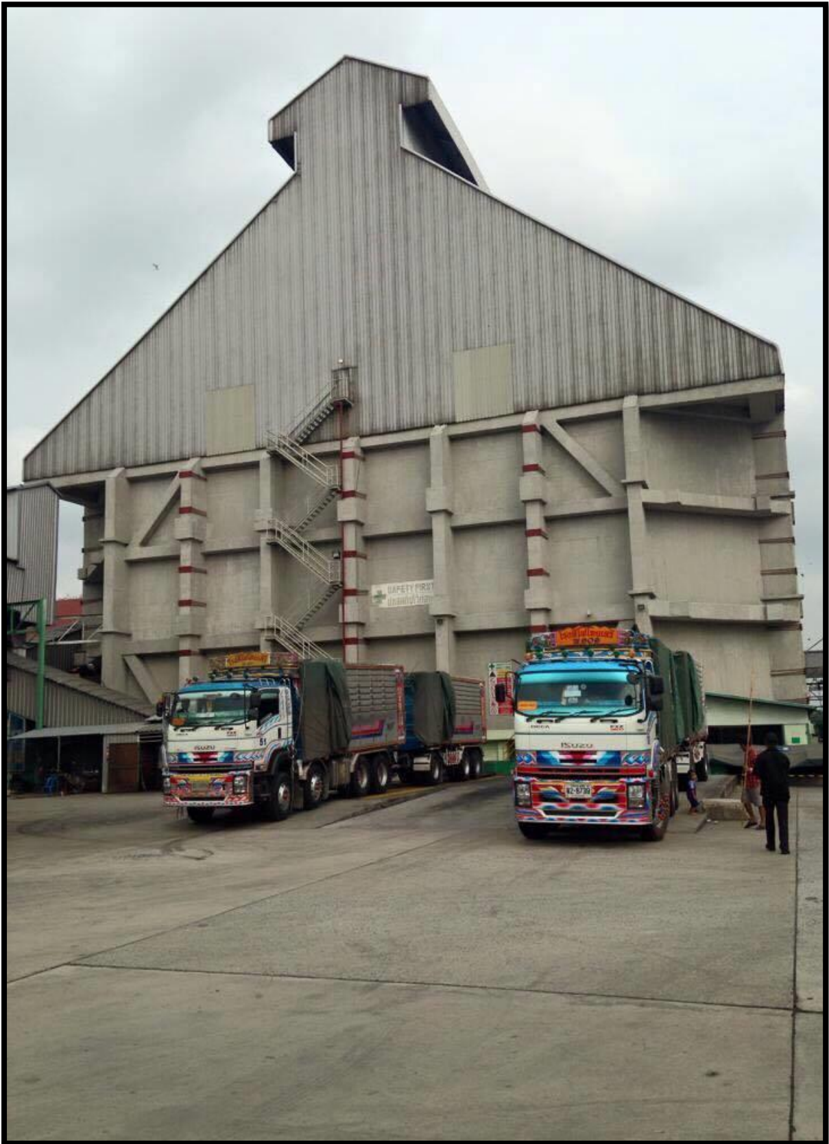
Warehouse rear view
